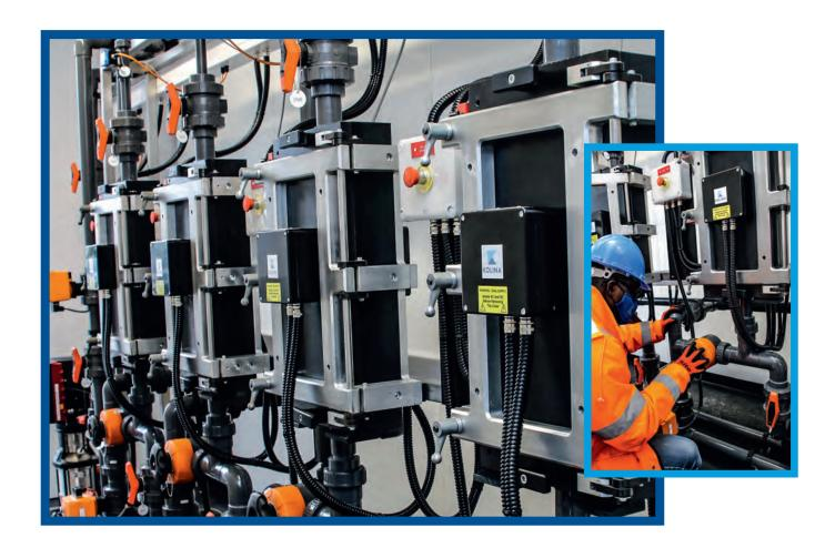
Kolina's EC technology offers a greener alternative to chemical dosing for removal of phosphorus; it generates coagulant ferric ion species through an electrochemical reaction in the EC cells between passed current and sacrificial electrodes. The generated coagulant ions have a utilisation efficiency of close to 100%, while dosed chemicals such as ferric sulphate and ferric chloride have utilisation efficiencies of between 28% and 34%.
